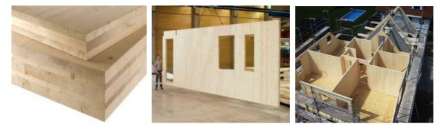
Figure 1, cross laminated timber
